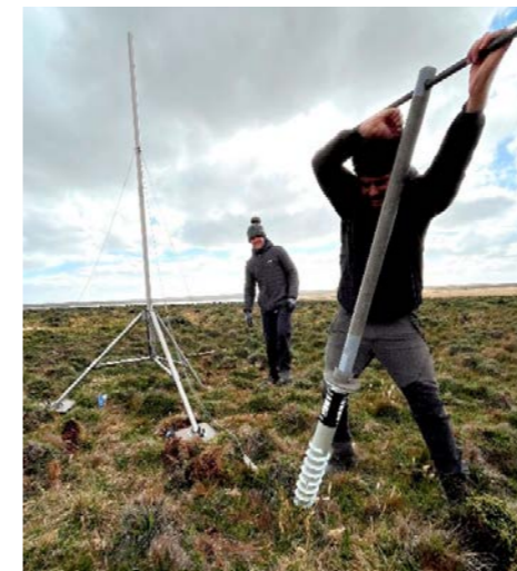
LEFT Ground anchor screws being installed to secure flux tower tripod against the typical high winds of the Falkland Islands; CENTRE Flux tower tripod with some units attached whilst survey work is carried out; RIGHT UKCEH team nearing completion of flux tower installation. Each tower took around three days to install.
