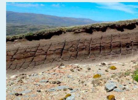
Erosion can also occur on upland sites with the drying out and cracking through the depth of the peat profile.
