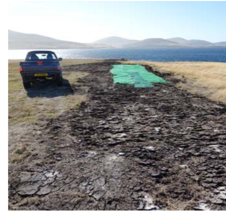
Work on the New island airstrip was completed. FALKLANDS CONSERVATION
