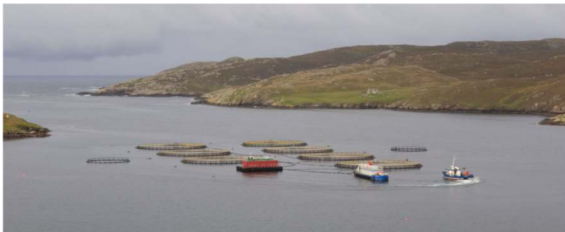
Figure 3: Example of net pen growout site (Shetland Isles) with feed barges and work boat. Surface components of the mooring system can be seen. The pens are covered with bird netting. Image – Andrew Schneider.
